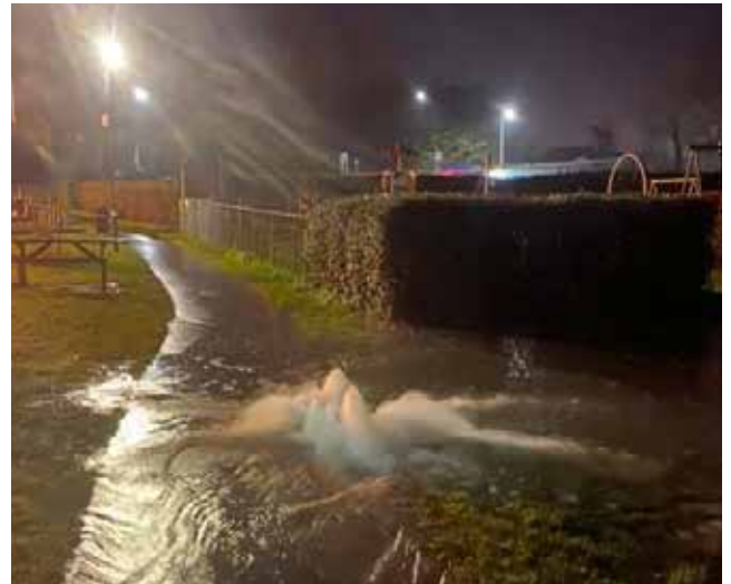
Water gushing up from drains by the play area
