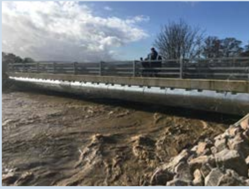
Spring Gardens bridge, Feb 2020
