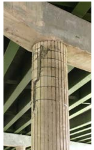
It's spalling...
