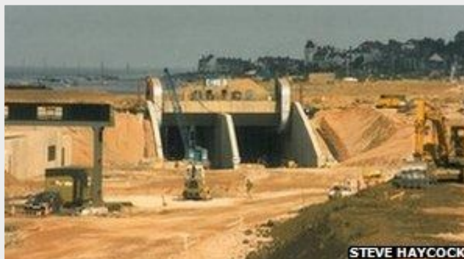
The Conwy Tunnel in construction
