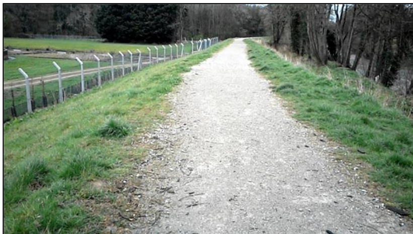
Figure 27: St Asaph STW Embankment Visual Inspection 2019 (NRW)
