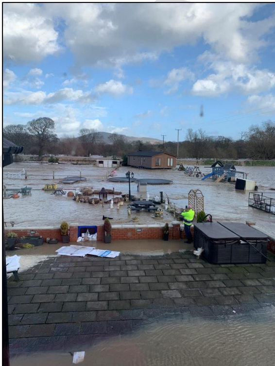
Figure 32: Extensive embankment overtopping at Dol Afon (Elwy resident, 2020)
