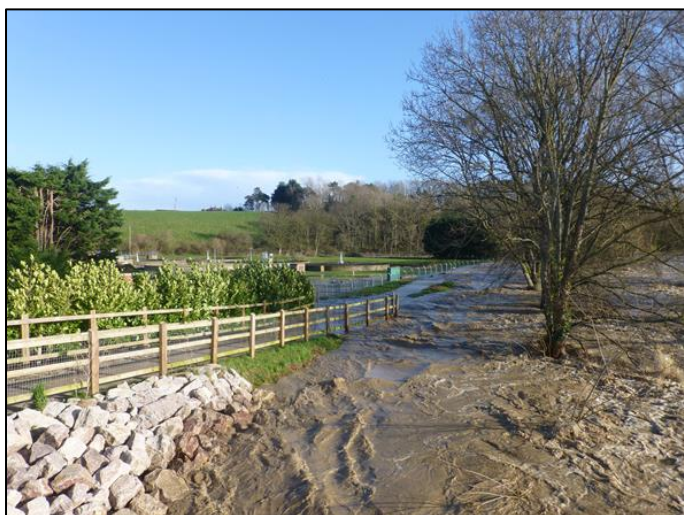
Figure 45: Water levels looking u/s from SGB (Resident photo)
