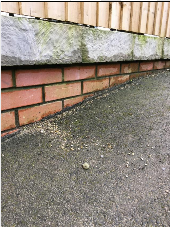
Figure 90: River gravel deposit on Foxons Ramp (NRW, 2020)
