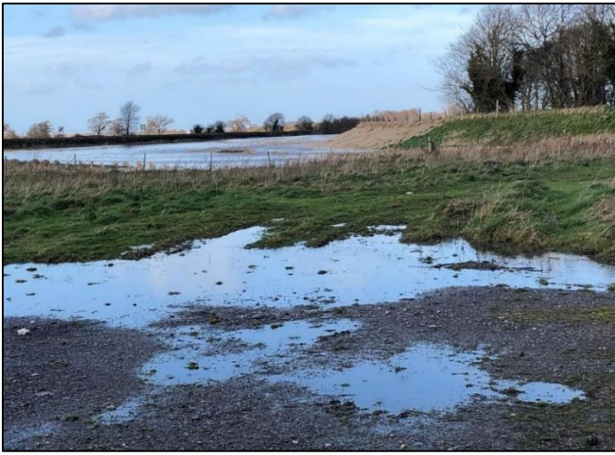
Figure 34: Phase 1 - Extensive overtopping at EMB1500412 (NRW 2020)
