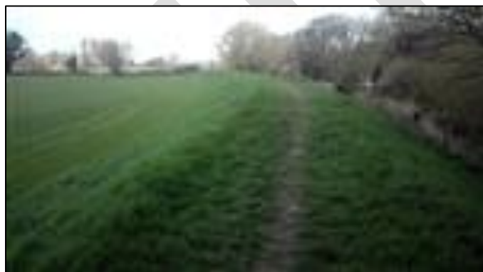
Figure 22: Elwy Fishermans Bridge Embankment (NRW, 2019)
