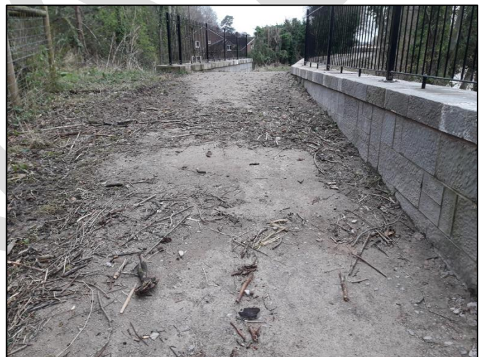
Figure 111: Wrack marks at Pont Begard wall (NRW, 2020)
