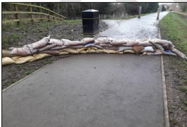
Figure 52: Sandbags placed at Roe Parc by residents looking downstream (NRW, 2020)
