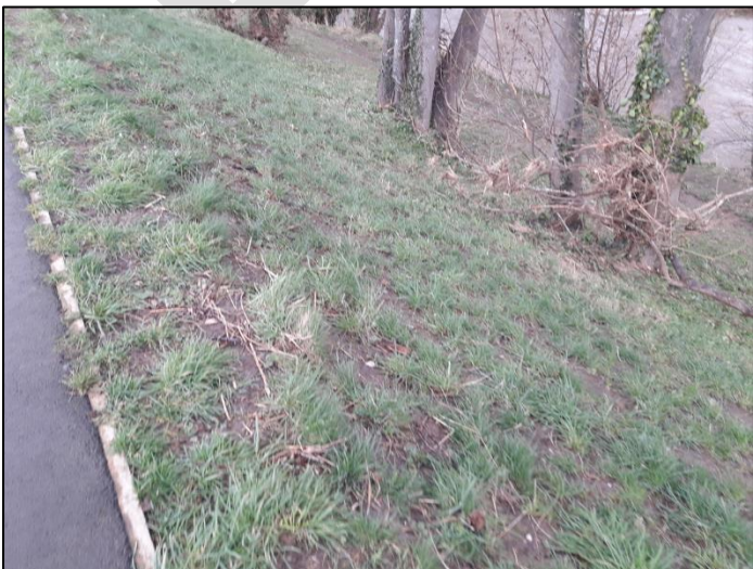
Figure 101: Wrack marks u/s library wall (NRW, 2020)
