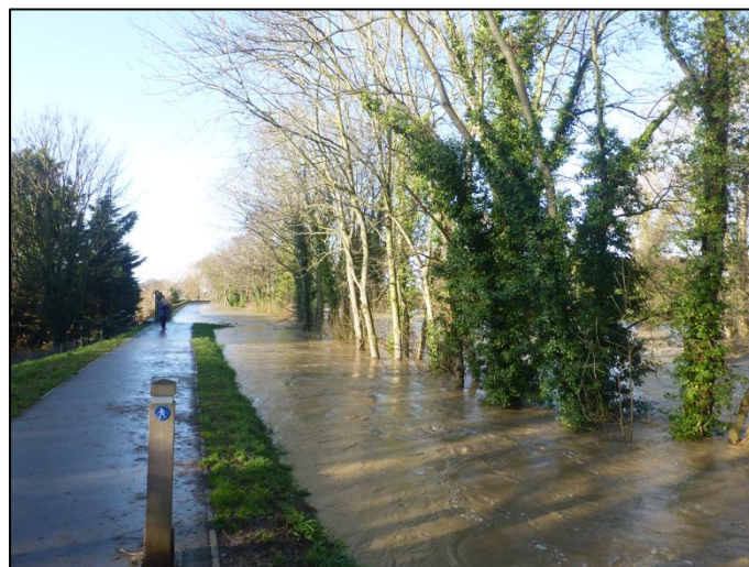
Figure 54: Water levels at u/s end of Roe Parc Wall (Resident photo)
