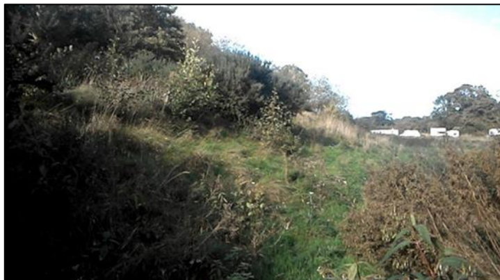
Figure 23: Elwy Mount Embankment (NRW, 2019)
