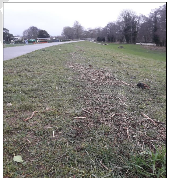
Figure 106: Wrack mark common emb (NRW, 2020)
