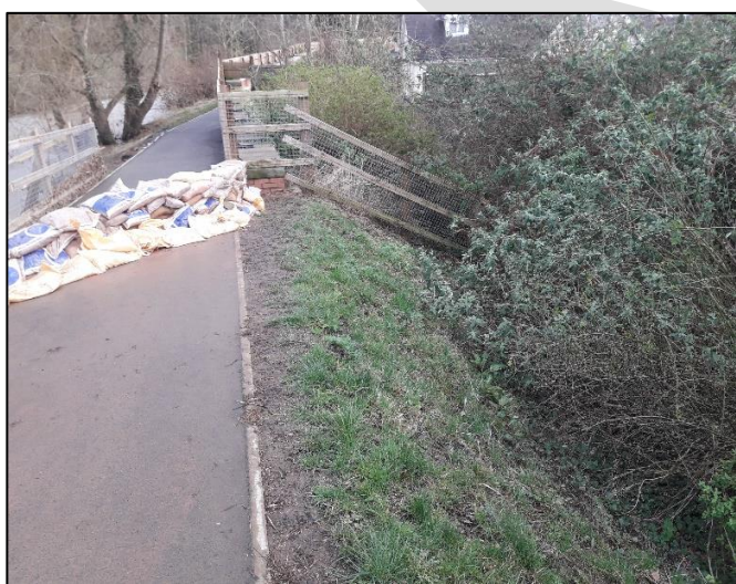
Figure 56: Sandbags placed at Roe Parc wall by residents (NRW, 2020)
