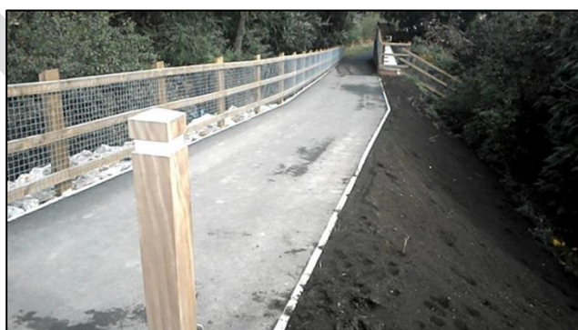
Figure 24: Roe Parc wall & embankment transition post-construction (NRW, 2018)
