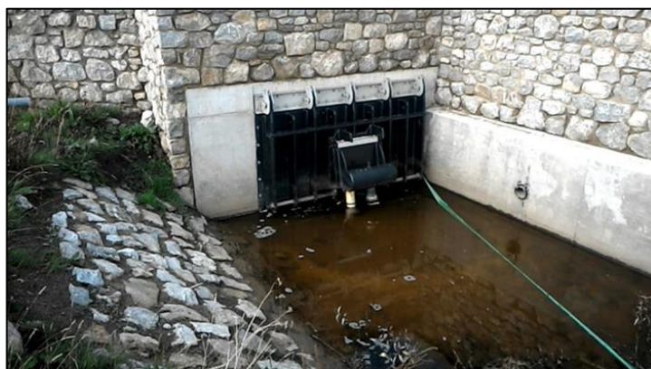
Figure 29: Glascoed Stream non-return flap (NRW, 2019)
