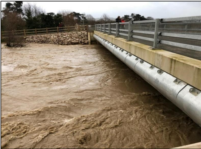
Figure 97: River levels 09-02-2020 compared to bridge deck (NRW, 2020)
