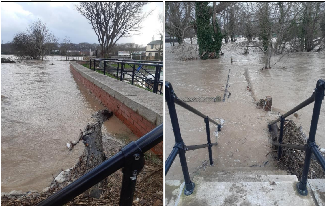
Figure 119: Water levels at the U/S end of Ruby Terrace (NRW, 2020)
