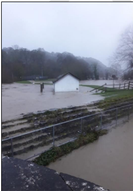
Figure 77: Overtopping Llanfair TH Elwy embankments back into the Elwy (Resident photo)
