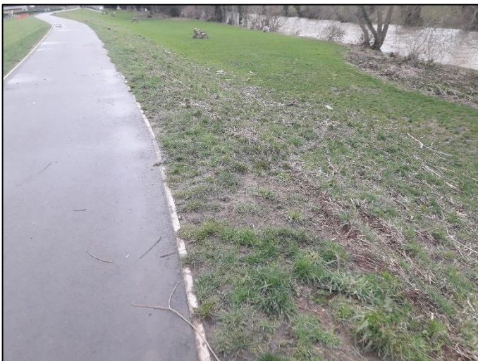
Figure 112: Wrack mark common emb (NRW, 2020)
