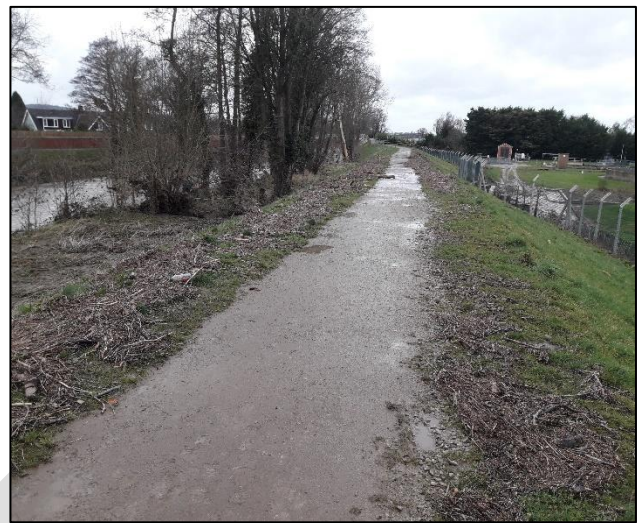
Figure 47: Line of wrack on RB STW emb (NRW, 2020)
