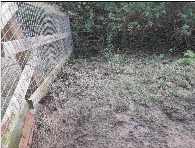
Figure 93: Location of overtopping Roe Parc Wall (NRW, 2020)
