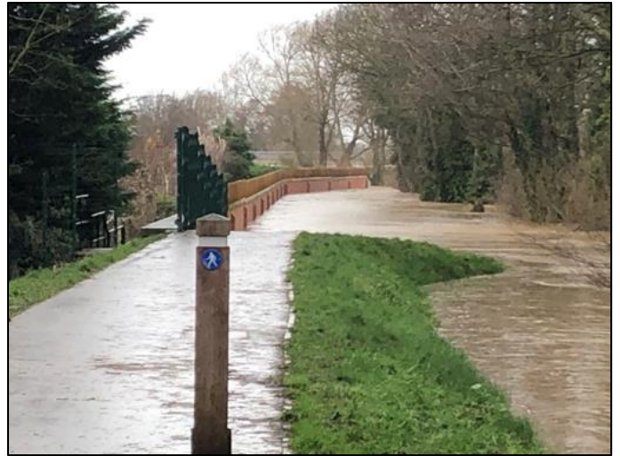
Figure 116: Prior to peak water levels at u/s end of Roe Parc Wall (Resident photo)
