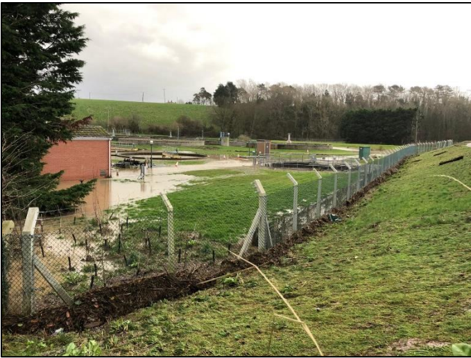
Figure 100: Post event debris (Resident photo)
