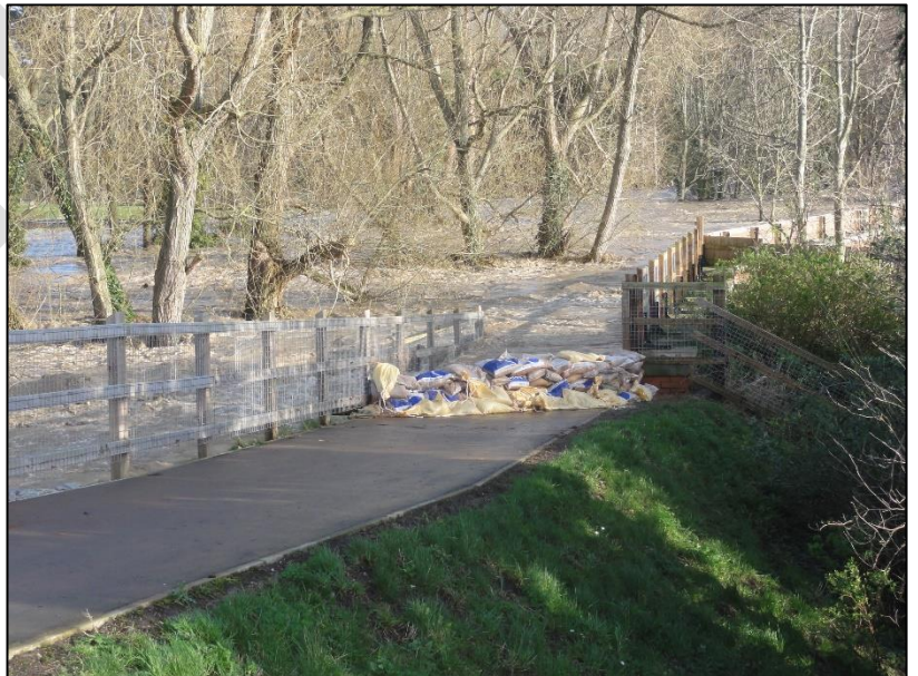
Figure 89: Sandbags deployed at Roe Parc Wall (Resident photo, 2020)
