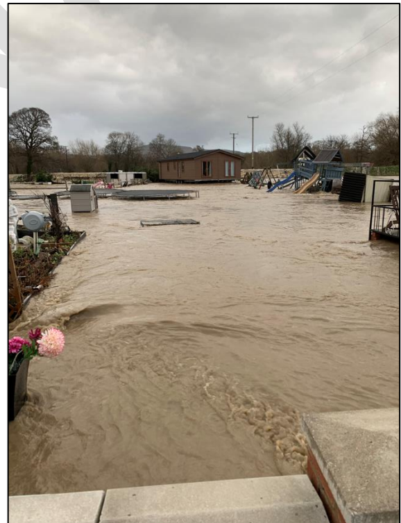
Figure 33: Extensive embankment overtopping at Dol Afon (Elwy resident, 2020)
