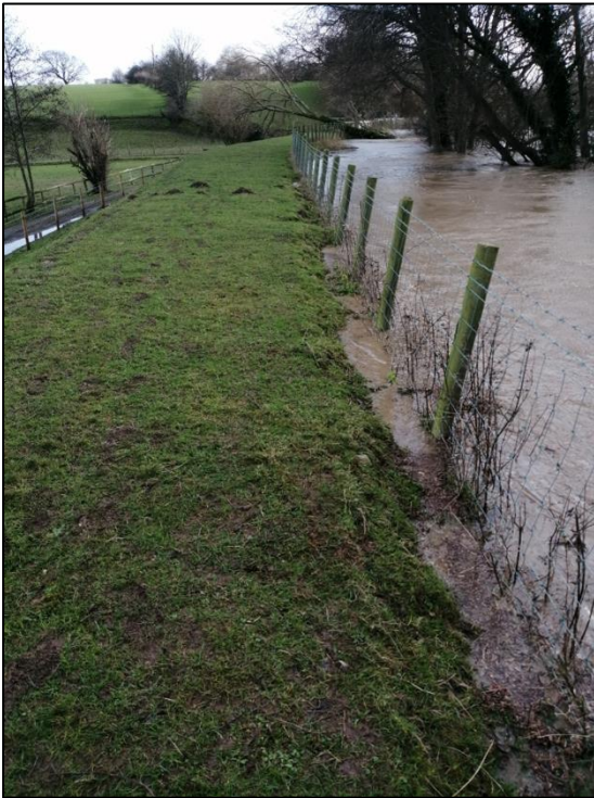
Figure 88: River levels d/s of fishermans bridge (NRW, 2020)
