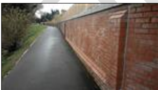
Figure 25: Roe Parc Wall (NRW, 2019)
