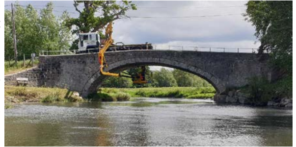
Inspecting the bridge before the collapse; note the asymmetrical arch
