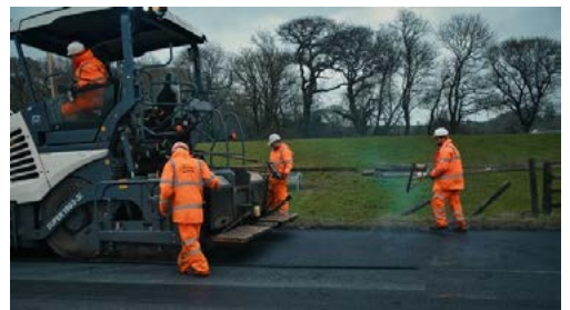
A 1.4-mile stretch of road between Cardigan and Aberystwyth has been re-paved using 107,000 recycled disposable nappies. Fibre from the nappies is added to the bitumen that glues together asphalt road surfaces. (images: Pura)
