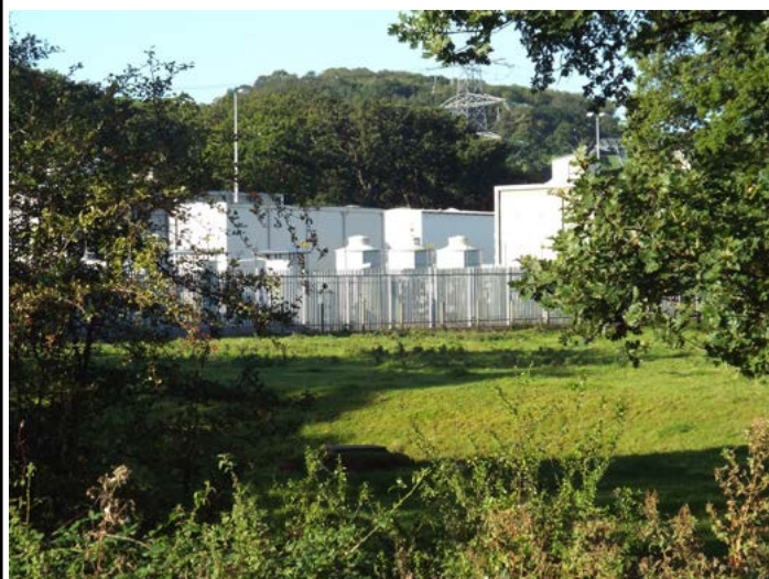
The well-concealed "Bodelwyddan" substation
