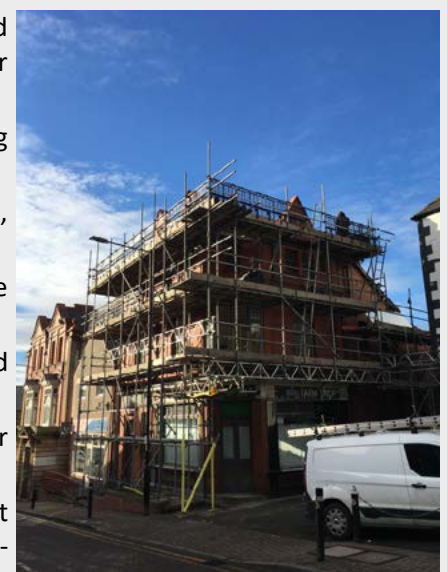
Work starts on the roof at the Central Buildings, the former Farm shop.
