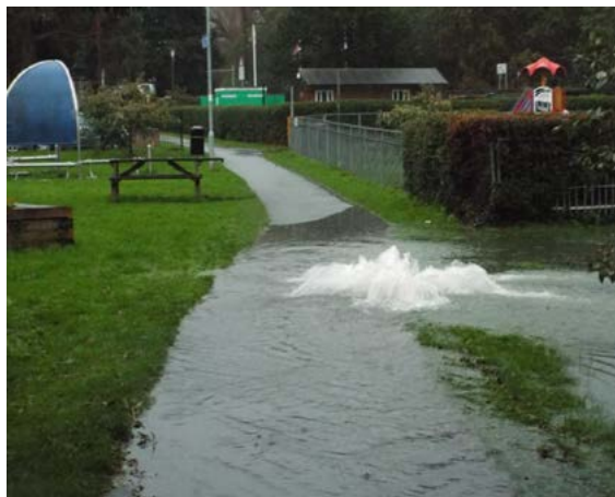
Water fountains out from the manhole
