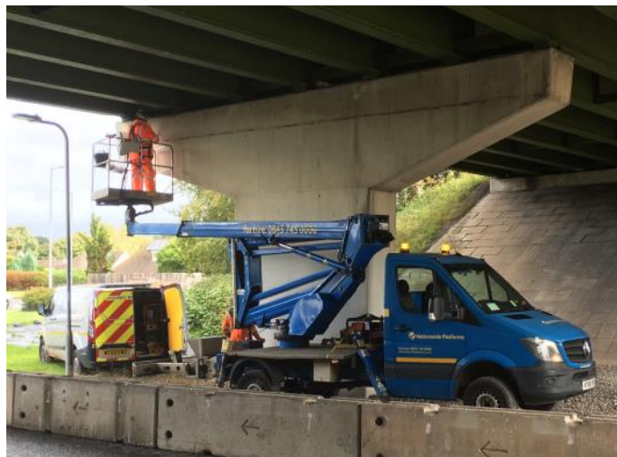
Taking samples of dust and concrete for lab analysis—at the roundabout
